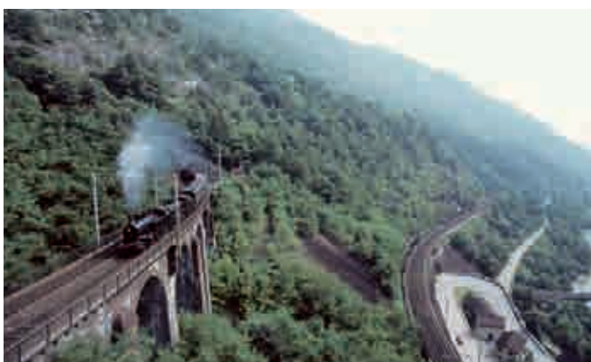
Gotthard Railway > Biaschina south ramp with three track levels. Photograph 1997. H.P. Bärtschi
