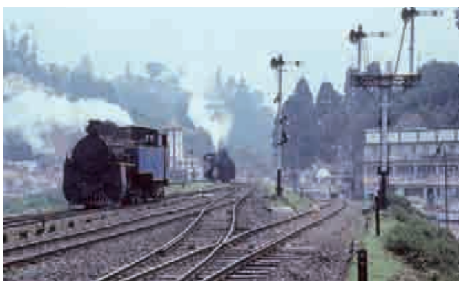
Nilgiri Railway > Transition from cog wheel to adhesion railway at Coonoor. Photograph 1988. H.P. Bärtschi
