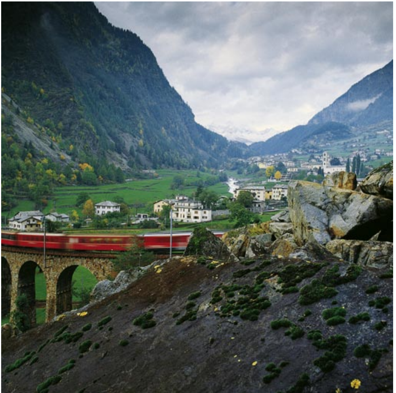
Bernina line > The Bernina railway on the circular viaduct at Brusio. R. Pedetti
