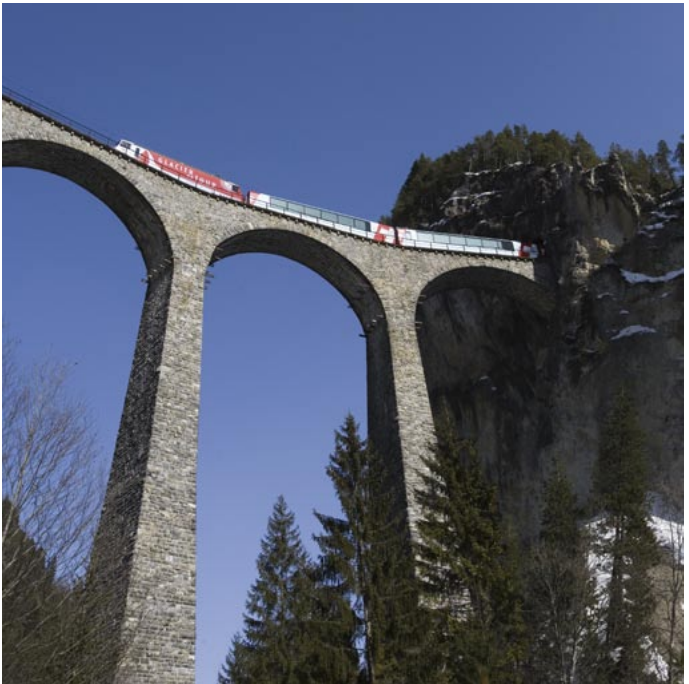
Albula line > The 65 m high Landwasser Viaduct, the most spectacular engineering structure between Thusis and St. Moritz. A. Badrutt/Rhaetian Railway
