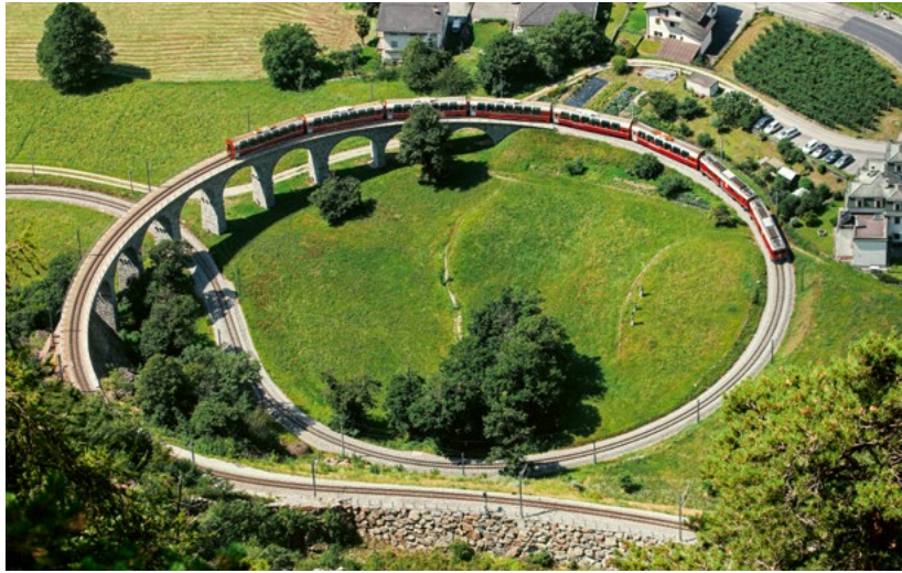
Circular Viaduct/Brusio, 780 m a.s.l. 11
